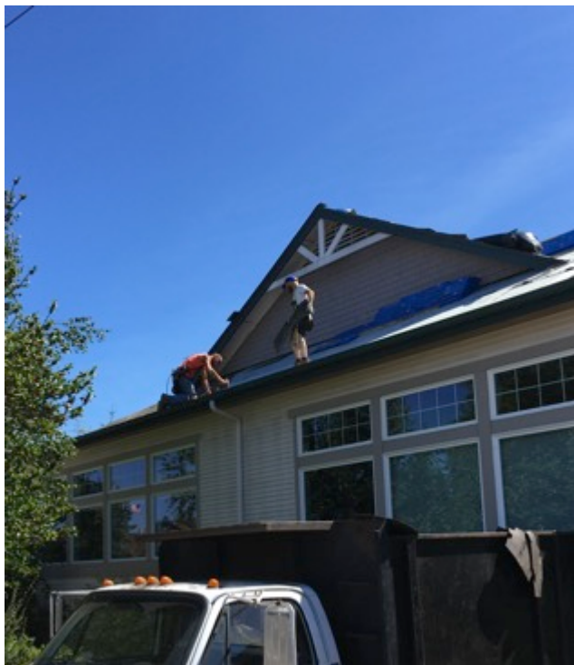
Last Phase of Re-roofing Project Complete
